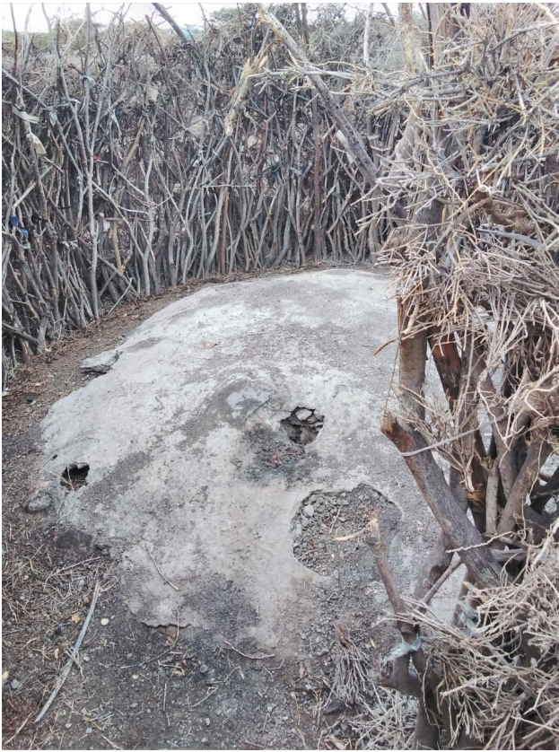
Pit latrine that Mama Kaikor Nakali constructed using locally available materials.
