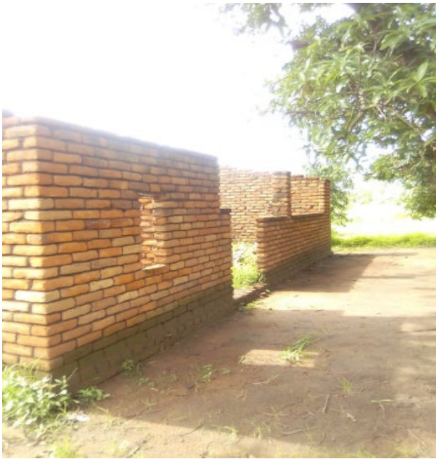
Msonthe village clinic construction project in progress, now at roofing stage.
